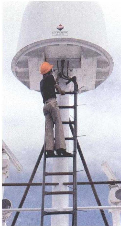
A technician from Satellite Services, Inc., of Houston, Texas, performing antenna radome installation on board the seismic vessel Acadian Commander in the Houston Ship Channel. Photo by William J. Megna.
